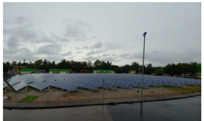
The Solar Farm constructed at Siu Ho Wan Sewage Treatment
